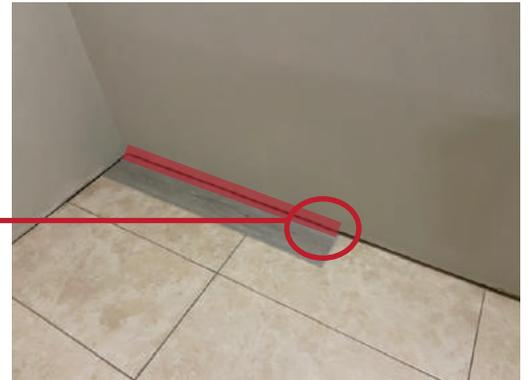
3. Begin by laying the first piece on the left side, with the groove of the long edge facing towards you.
